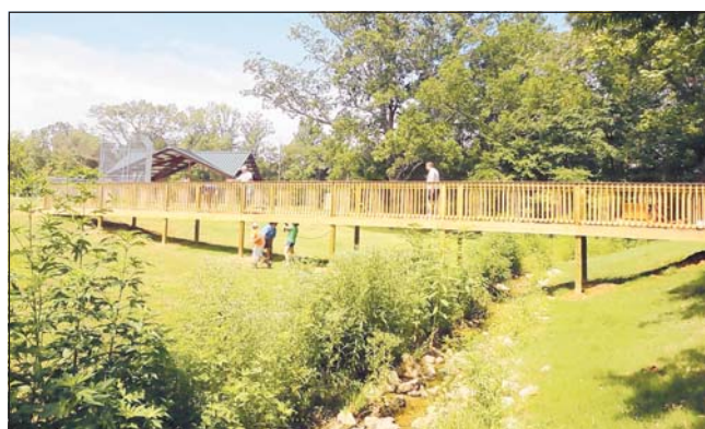
It took Allan Sisson and 33 volunteers three weeks to finish the 100-foot long wooden bridge. The bridge, which was completed in mid-August, was part of Sisson's Eagle Scout project.
